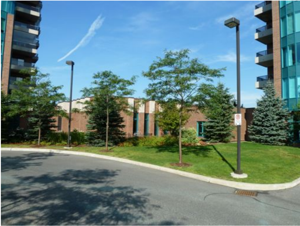
1. General view of the Shared pool building between OSCCC 667 and OCSCC 769.
