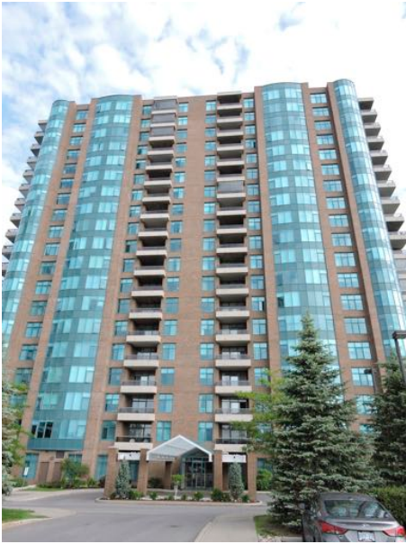
Photo 1 General view of the OCSCC 769.
