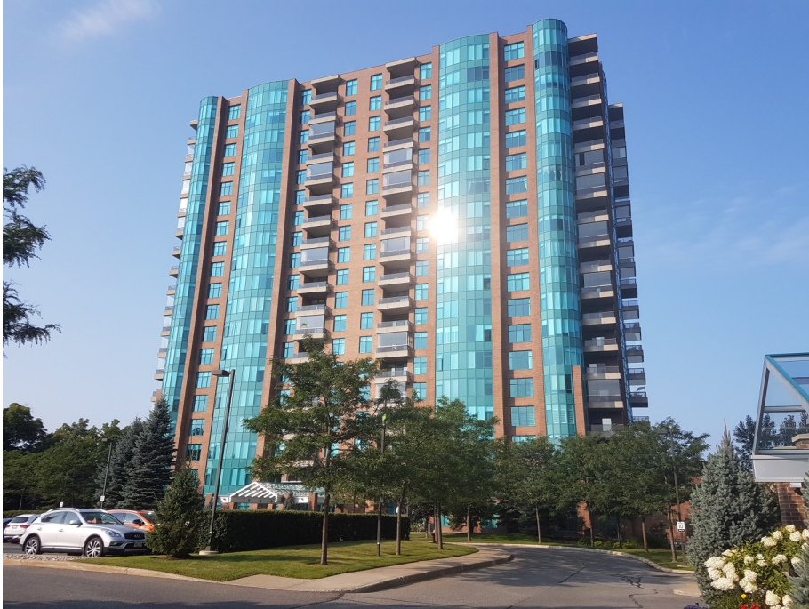
1. Partial front elevation of OCSCC 769
